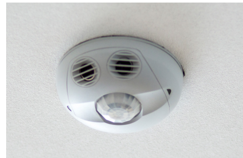
A lighting vacancy sensor saves energy by automatically turning off lights when a room is empty.
