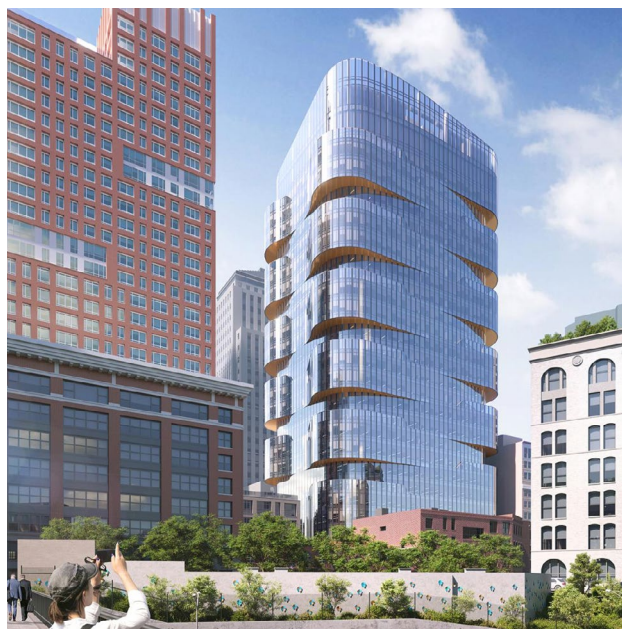
380 STUART STREET- DESIGNED IN ALIGNMENT WITH BOSTON'S PROGRESSIVE GREEN BUILDING AND CARBON-NEUTRAL GOALS. PHOTO: CBT ARCHITECTS
