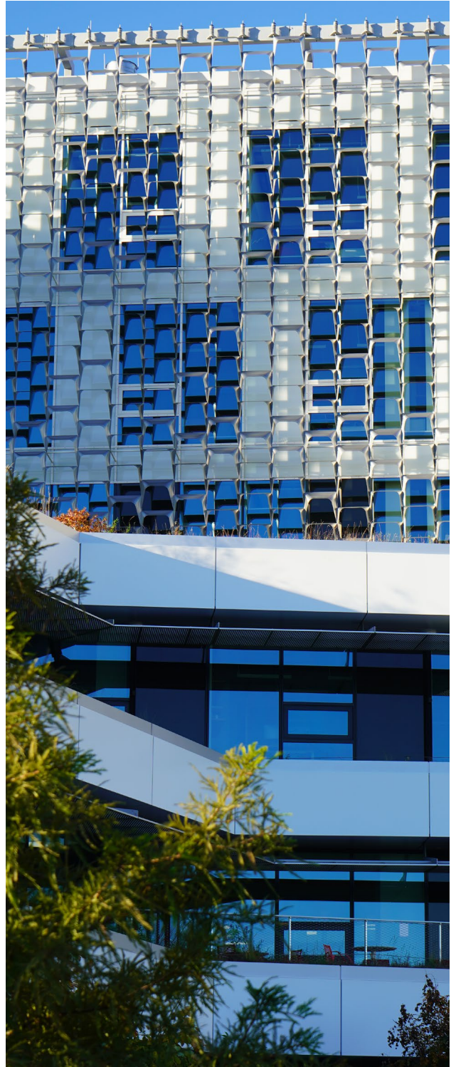
HARVARD UNIVERSITY SCIENCE AND ENGINEERING COMPLEX - NAMED ONE OF THE HEALTHIEST, MOST SUSTAINABLE, AND ENERGY-EFFICIENT LABORATORY BUILDINGS IN THE WORLD
