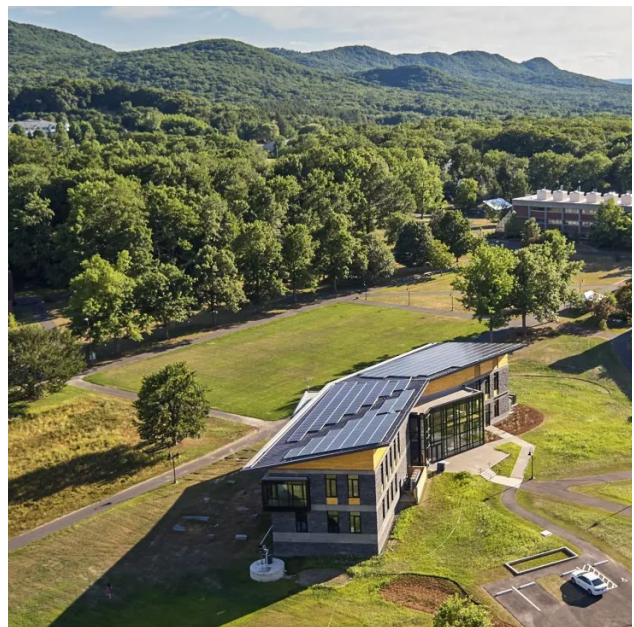
R.W. KERN CENTER - THE LARGEST LIVING CERTIFIED HIGHER-EDUCATION PROJECT IN THE WORLD AT THE TIME OF ITS COMPLETION. PHOTO: BRUNER/COTT ARCHITECTS
