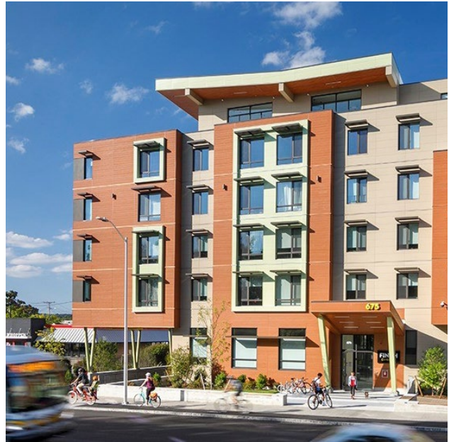
FINCH CAMBRIDGE - THE FIRST AFFORDABLE PASSIVE HOUSE BUILDING IN MASSACHUSETTS. CAMBRIDGE, MA. PHOTO: ROBERT UMENHOFER
