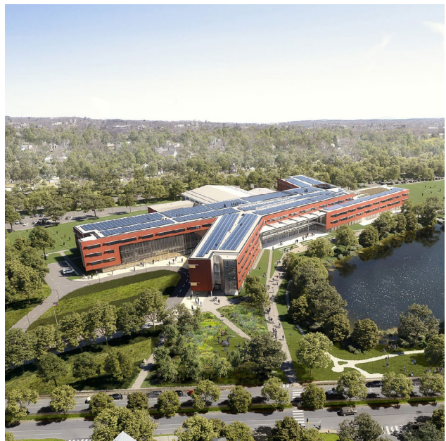
BELMONT MIDDLE & HIGH SCHOOL - 100% ELECTRIC WITH A GEOTHERMAL WELL HEAT PUMP SYSTEM TO PROVIDE HEATING AND COOLING TO THE BUILDING. PHOTO: PERKINS+WILL
