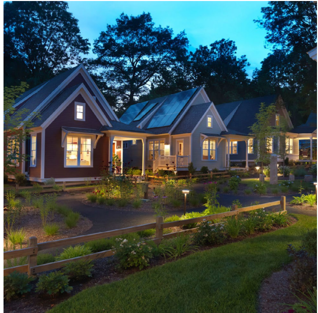
CONCORD RIVERWALK - WITH VERY TIGHT BUILDING ENVELOPES, EACH COTTAGE ONLY USES AS MUCH ENERGY AS CAN BE PROVIDED BY ON-SITE SOLAR. PHOTO: UNION STUDIO ARCHITECTURE
