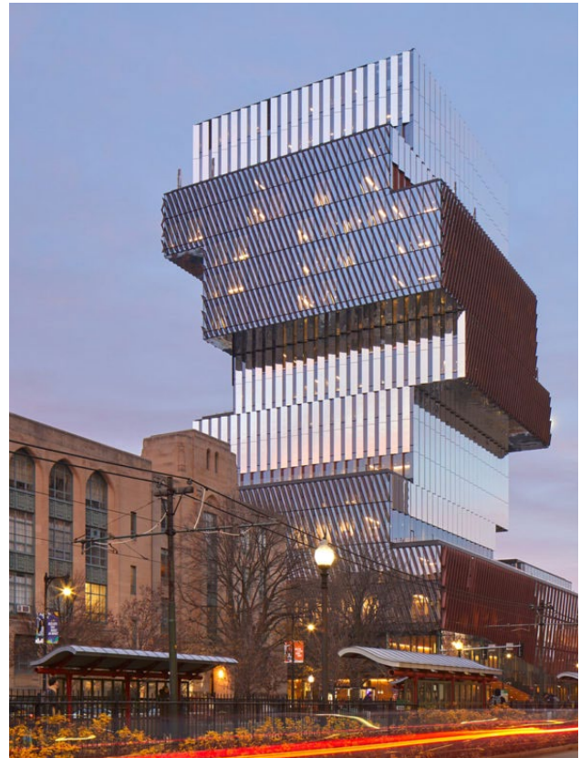
BOSTON UNIVERSITY, CENTER FOR COMPUTING & DATA SCIENCES - THE LARGEST NET ZERO ENERGY BUILDING IN BOSTON. PHOTO: TOM ARBAN
