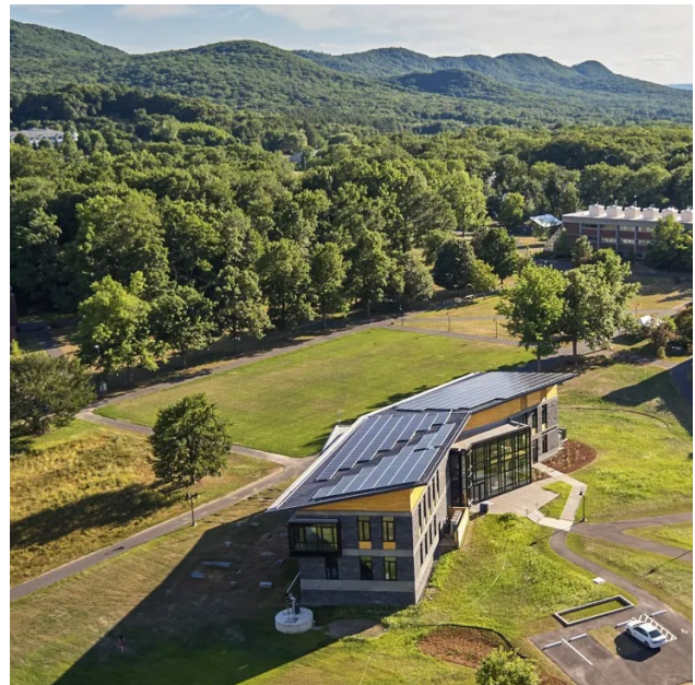
R.W. KERN CENTER- THE LARGEST LIVING CERTIFIED HIGHER-EDUCATION PROJECT IN THE WORLD AT THE TIME OF ITS COMPLETION. AMHERST, MA. PHOTO: BRUNER/COTT ARCHITECTS
