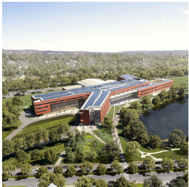
BELMONT MIDDLE & HIGH SCHOOL - 100% ELECTRIC WITH A GEOTHERMAL WELL HEAT PUMP SYSTEM TO PROVIDE HEATING AND COOLING TO THE BUILDING. BELMONT, MA. PHOTO: PERKINS+WILL
