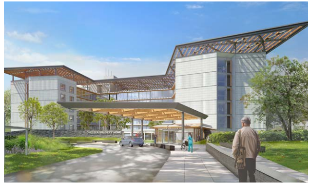
The Chelsea Soldiers' Home New Community Living Center will be a 236,000 sf assisted living facility, designed to achieve Class D Zero Net Energy with a predicted site EUI below 60 kBtu/sf*yr. Systems include: high-performing envelope, natural ventilation, geothermal, water-source heat pumps, and a 0.7MW PV array canopy above the roof. This was achieved at a construction cost premium of 0.1% of project cost. With the anticipated $750,000 in incentives and grants, it costs less to build than the business as usual case. Owner: DCAMM, Architect: Payette, Mechanical Engineer: BR+A. Image credit: Payette.
