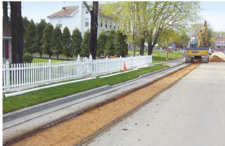
Vacuum sewer installation causes minimal disruption to neighborhoods. Trenches are shallower, less excavation is required and streets can remain open to traffic.
